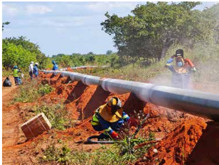
Ntorya-Madimba natural gas pipeline
