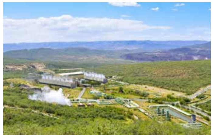
Olkaria IV Geothermal Power Plant Bridge
