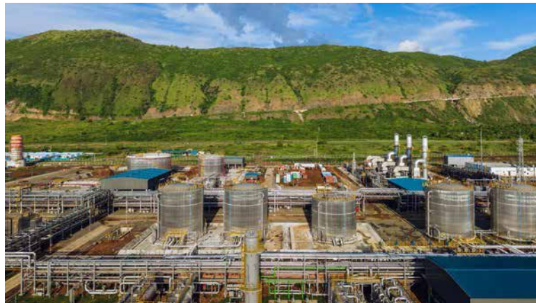
Kingfisher Central Processing Facility (40,000 BOPD): From Resource Discovery to Commercial Oil Production
