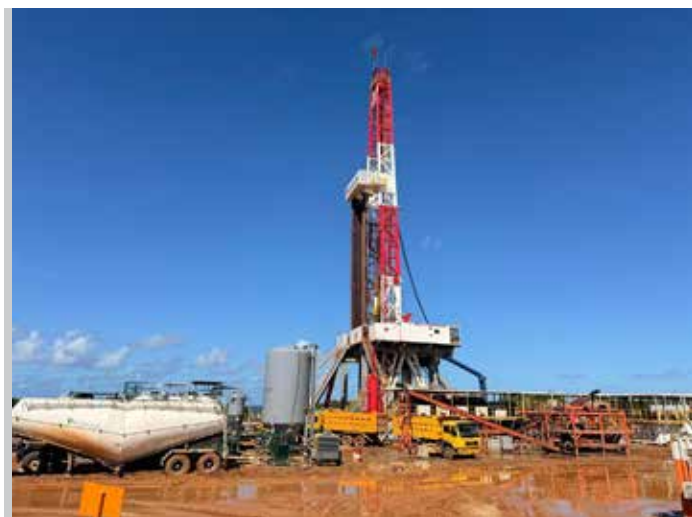
Drilling of production well in Mnazi Bay field
