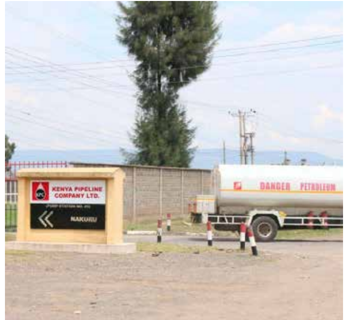
KPC Pump Station No. 25 in Nakuru
