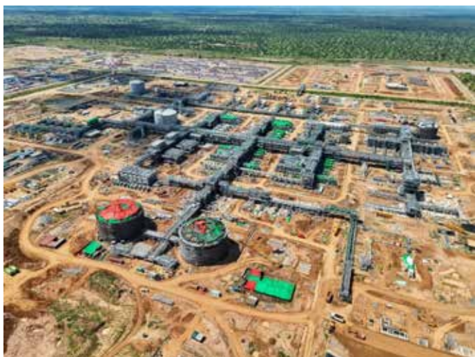
Aerial View of the Tilenga Central Processing Facility (CPF) in the Albertine Graben
