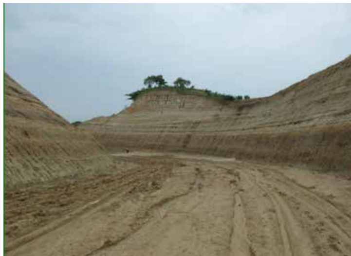
Kibuku Road Cut exposure during construction in June 2011
